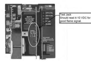
Flame signal strength can be checked by removing the red cover from the Fireye Chassis and reading the DC voltage across the test jacks located on the amplifier card. A reading of 4 to 10 VDC indicates a good flame signal. Holes may also be drilled in front cover to allow for measurements. See Fireye instruction manual MC-5000 for additional information.
